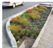
Curb extension with planted swale that captures stormwater from the gutter.
